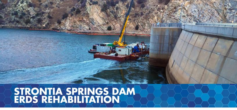
The Strontia Springs Dam reservoir's emergency reservoir drawdown system (ERDS) rapidly releases water in an emergency scenario through a 50ft. long tunnel that runs through the base of the dam. The thrust nut on the ERDS control gate was damaged and required replacement, 200ft. below the reservoir's surface. Denver Water selected Ballard as its CMAR partner to perform the necessary repairs.
