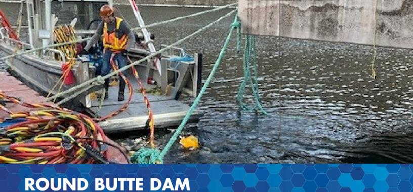
The existing Round Butte Dam power tunnel fill valve had not been used since 1972 and was operated by a hydraulic hand pump. To alleviate the risk of the valve not working, Ballard was retained to install two new valves to serve in its place. The existing valve was also removed and the line isolated with a blind flange.
