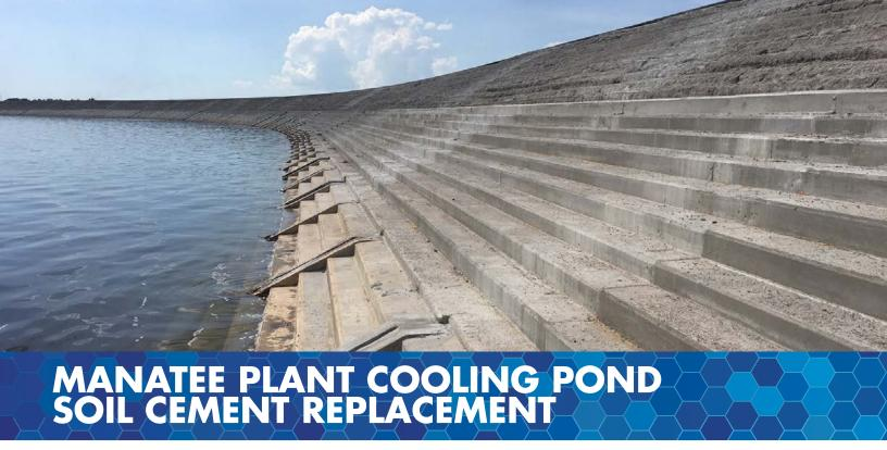
The Cooling Pond Soil Cement Replacement Project at the Florida Power and Light (FPL) Manatee Plant, located outside of Tampa, Florida, will extend the lifespan of the existing cooling pond and provide additional protection against severe tropical storms and hurricanes. The cooling pond is a key component of the power plant as it circulates and feeds cooling water to the plant's intake structures.
