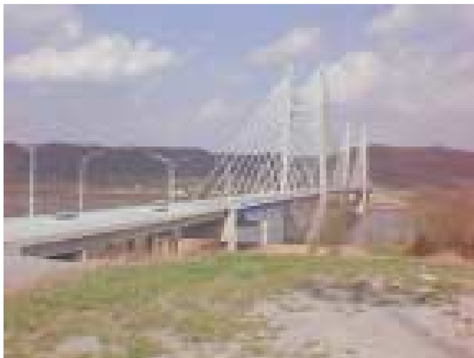
The William H. Harsha Bridge, designed by American Consulting Engineers and Michael Baker Corp., received the 2001 Grand Conceptor Award from the national competition sponsored by the American Consulting Engineers Council.
