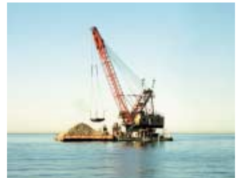
Derrick Barge "William F" placing rock on Hyperion Outfall.
