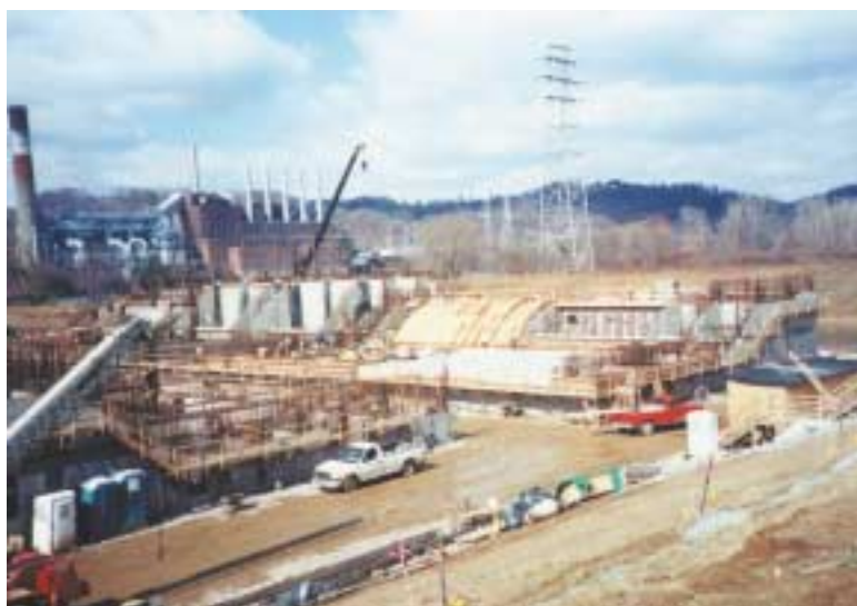
Segment One construction.
