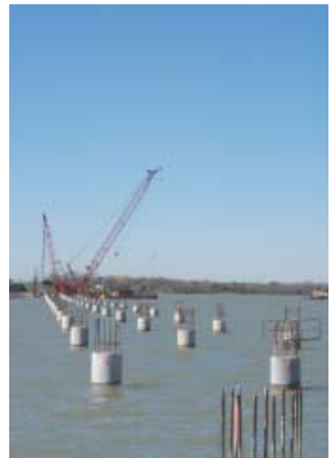
Drill shafts for westbound bridge, 147 completed, 117 remaining.
