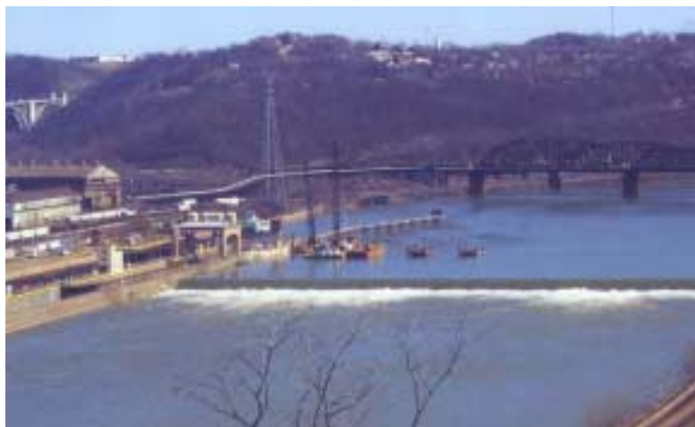
"In the wet construction" at Braddock Dam.
