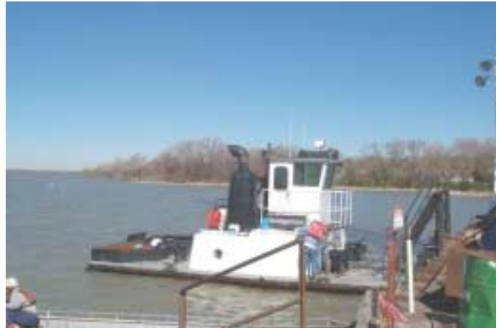
The "Bridgeman" prepares to take crane barge to work site.
