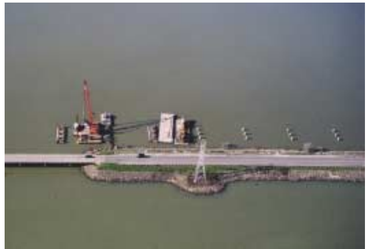
Shown is the Manitowac 3900 Drill Rig, Slurry Barge and Form Barges.
