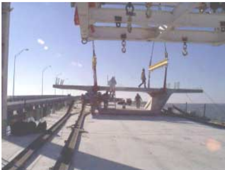
Placing a deck segment.
