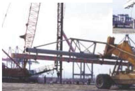
Handling and driving 30 ton concrete piles from shore.
