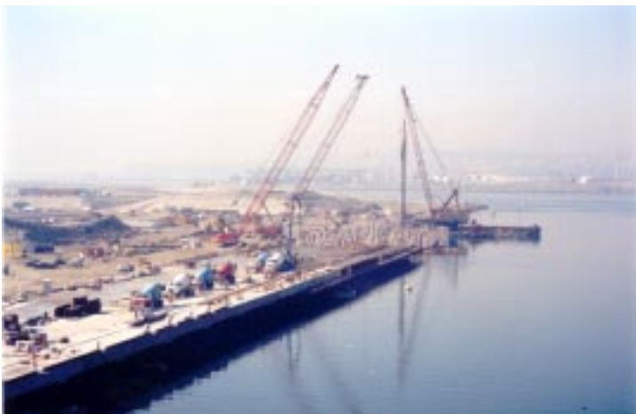
Wharf construction at Pier 400 is nearing completion in early March 2002.
