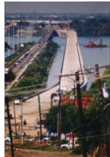
Completed westbound lane just prior to traffic switch.
