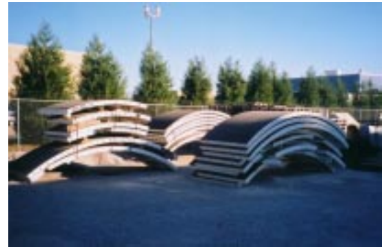
Fabrication of 32' diameter tunnel forms.
