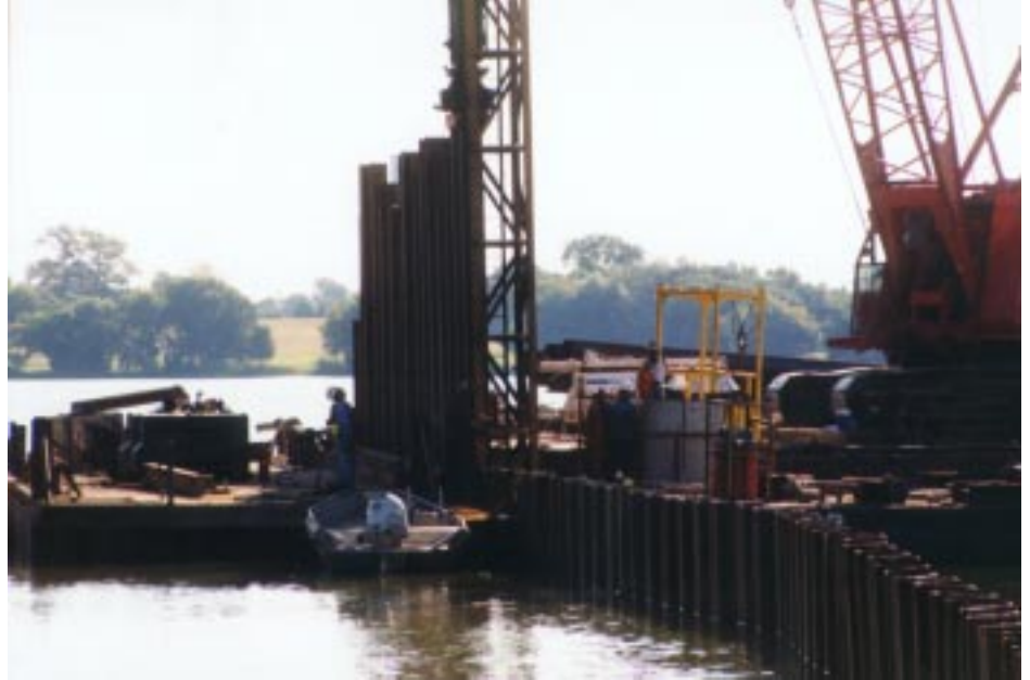
Installation of sheet pile wall.
