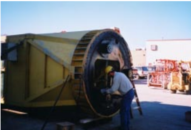
Repairs to the Liebherr 450 C.
