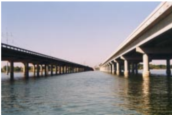
Looking west between old and new bridge.
