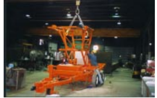
Repairs to a hydro platform.
