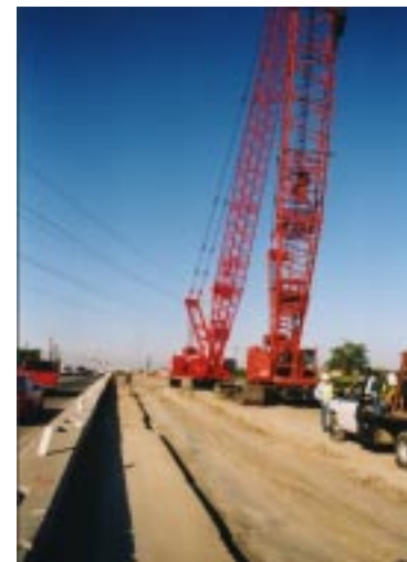
New 999 and 888 Manitowoc cranes ready to start eastbound lane.
