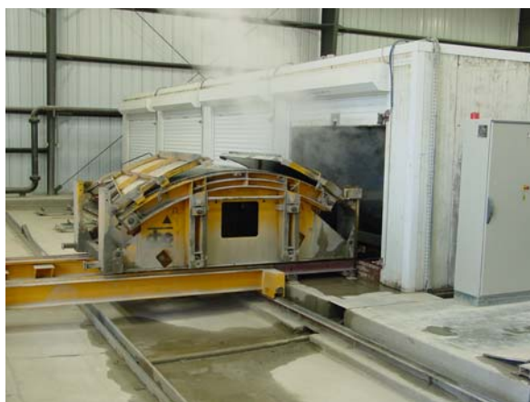
Freshly cast segment entering the steam curing room.
