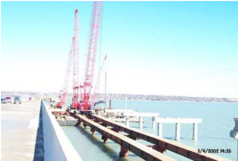
Eastbound bridge construction utilizing access trestle.
