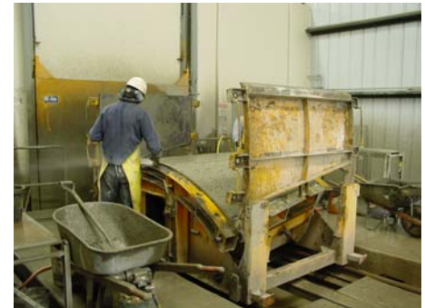
Finishing the segment extrados after concrete placement.
