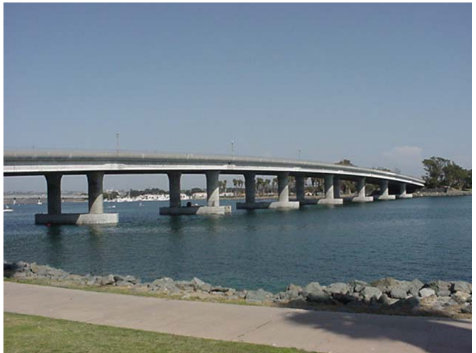
West Mission Bay Drive project near completion.
